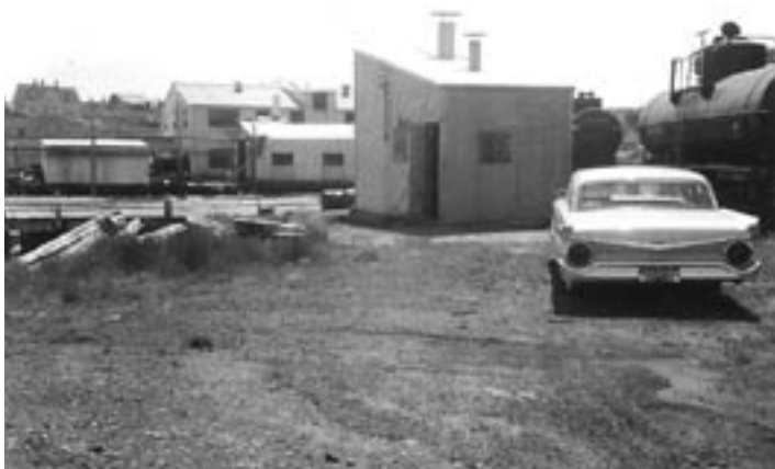
Sea Street 1950s shed containing a vertical tube boiler used in cold weather to supply steam to tank car heating coils, which warmed the soybean oil for ease in pumping.
